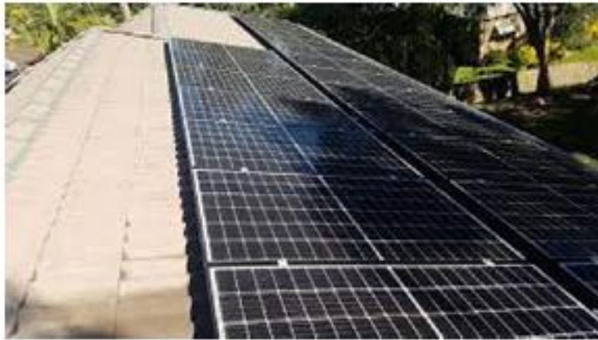
Fig. 16 shading on the solar PV cell
